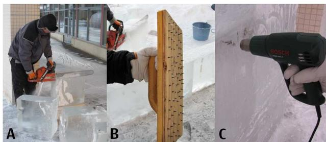
Figure 2. Useful tools for building an ice wall. A) Chain saw, B) tool for finishing, C) Hot air gun
