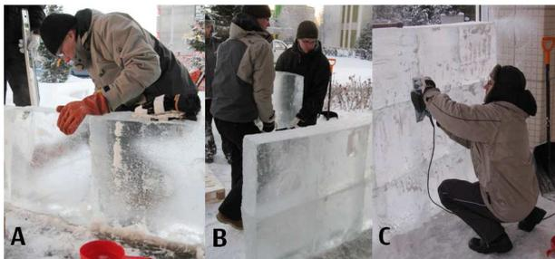
Figure 1. Building the screen. A) Jointing, B) Stacking, and C) Finishing the blocks
