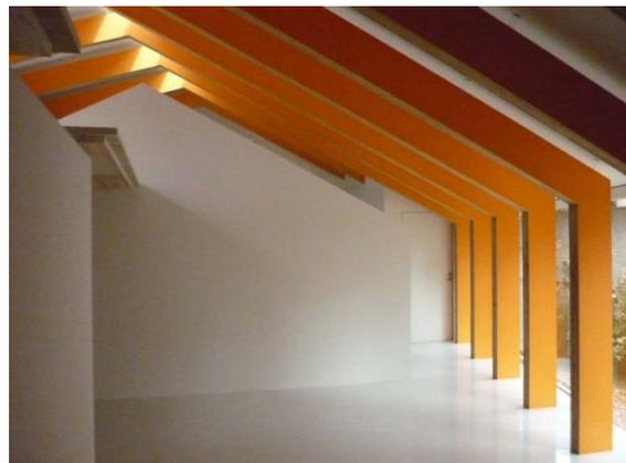
Figure 26: Ocha house is built on a skeleton of laminated wood frames.
