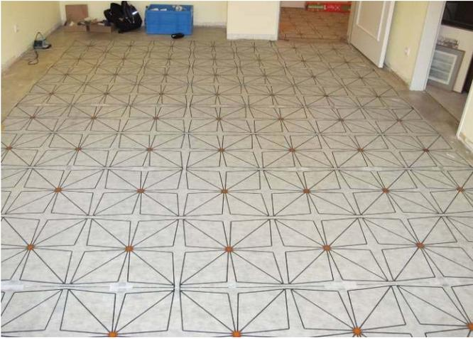
Fig. 1: Example of an installation of SensFloor under progress.
